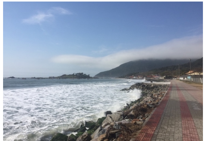
Figure 1: Existing seawall at Armação Beach.
