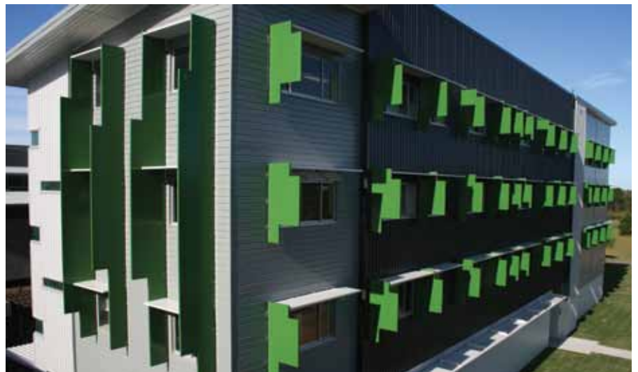
■ The $4.75 million science building was constructed over seven months in 2011.
